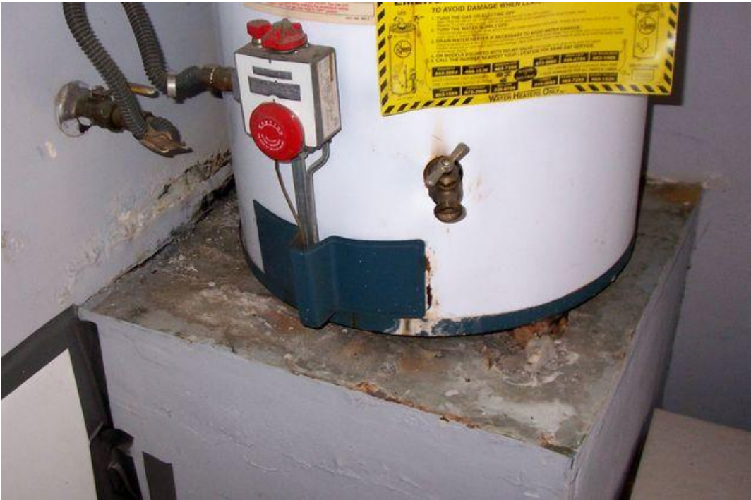
Although the age cannot be determined, this water heater is probably nearing the end of its effective life and should be replaced.
